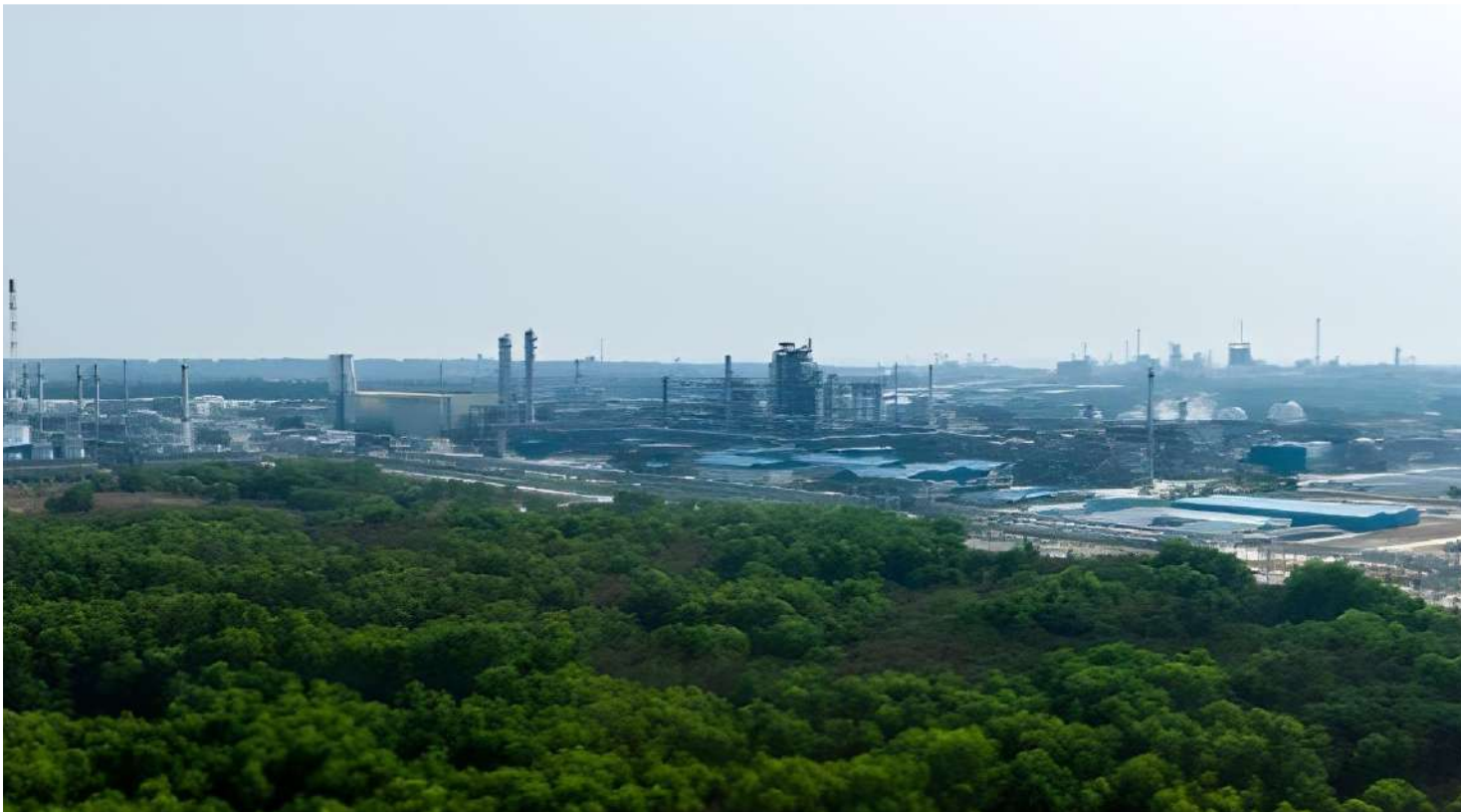
A petrochemical complex in Rayong province, Thailand. © EJF 2025. In Thailand and elsewhere, subsidies to petrochemical companies and plastics producers obscure the economic non-viability of single-use plastic production.
