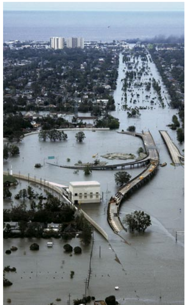
Flooding after Hurricane Katrina: one of 15 North Atlantic hurricanes in the record-breaking 2005 season.
